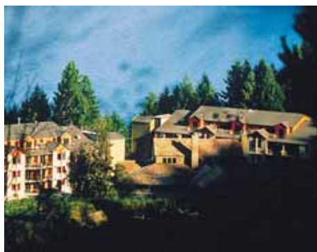
Heritage Hotel, Queenstown
