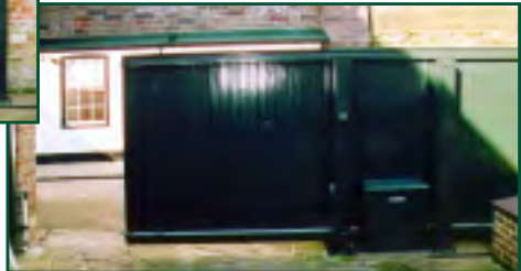
Rear view of Timber Sliding gate opening
