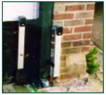
Closing posts with two pairs of photocells
