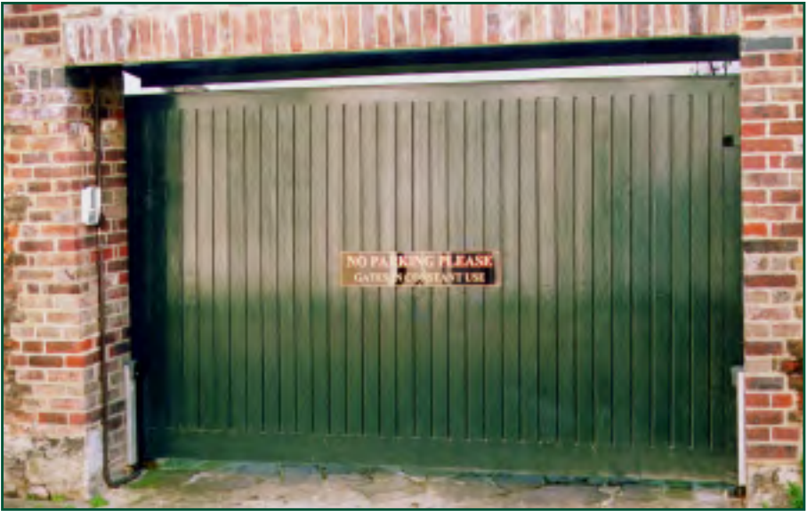
Front view of Timber Sliding gate
