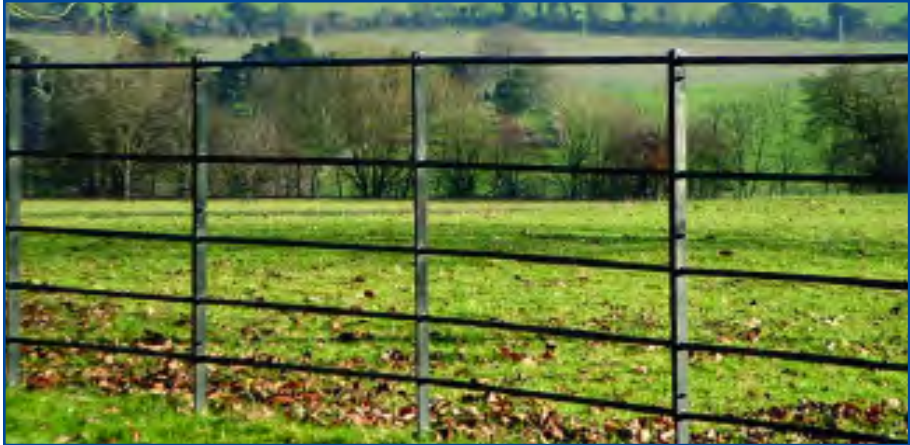
Estate Railings galvanized and polyester powder coated black
