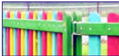
Pales, posts and gravel boards are all planed smooth with rounded edges to reduce splinters.
