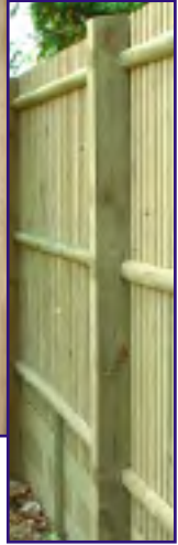
Rear view of fence showing centre stump and half round rails
