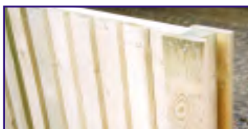
Panel and Jakpost, showing slot for panels
