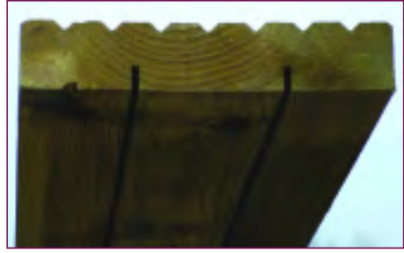
Detail of decking board profile showing the anti-slip grooves on top surface and the stress relief cuts on the bottom surface of boards to help avoid warping as boards expand and contract with the weather conditions.
