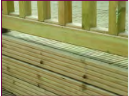
Close up showing decking boards used as edging for a neat and professional looking finish.
