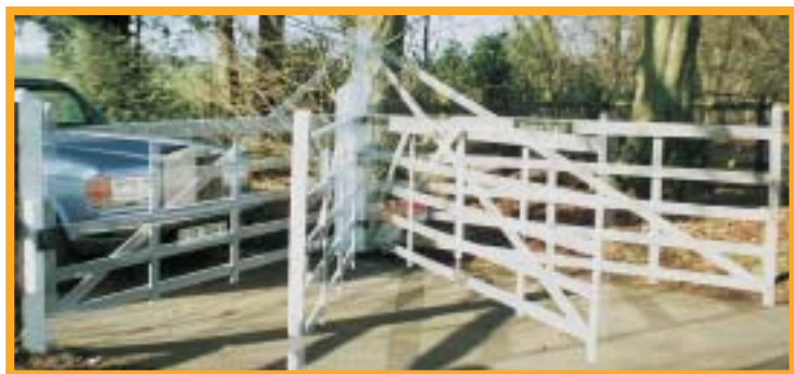
Automatic entrance gate in operation
