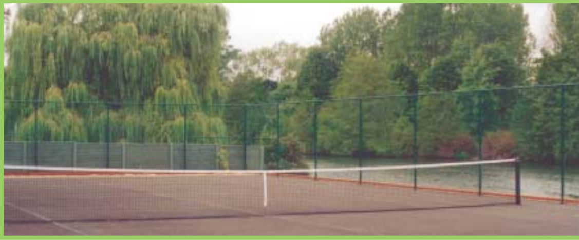
Tennis Court Surround galvanized with polyester powder coated finish clad with PVC coated chain link
