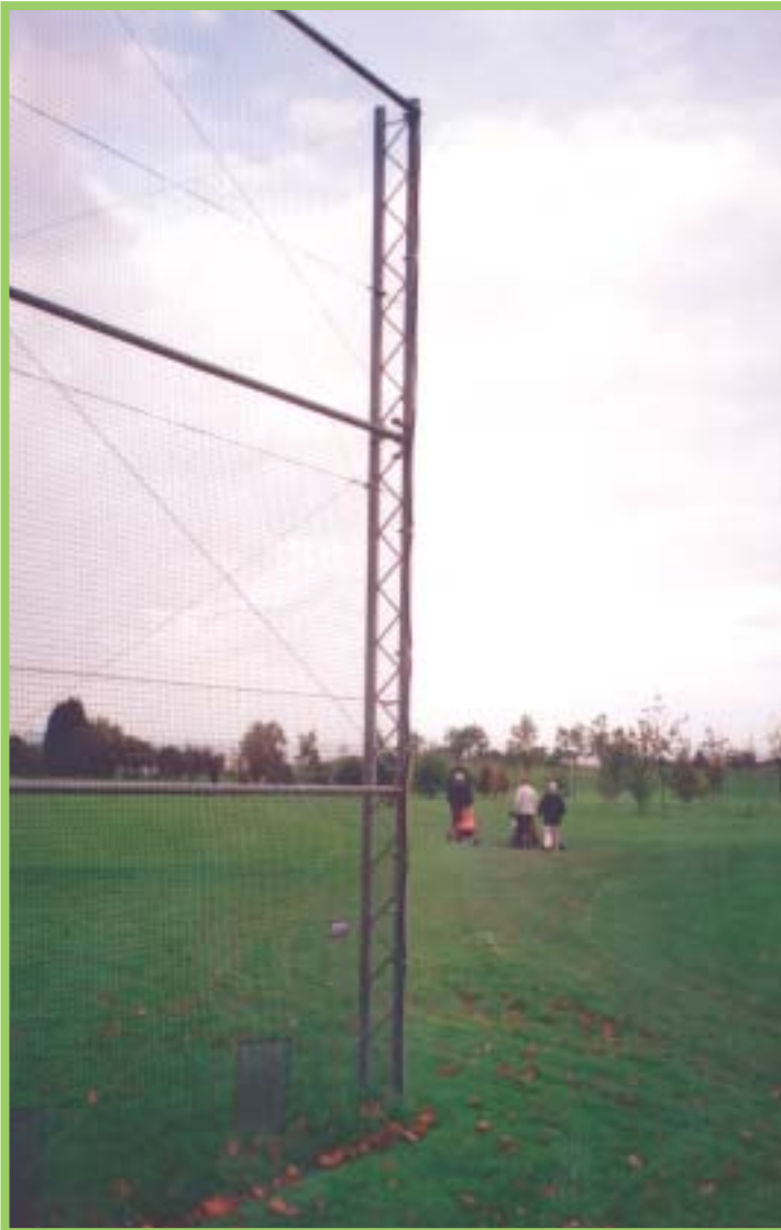
Ball-Stop Sports fencing employed on a golf course
