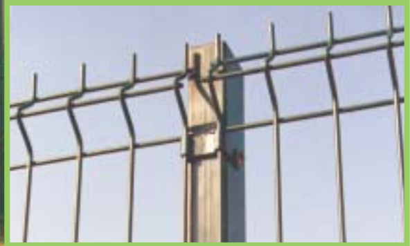
EuroGuard Regular panel and post detail with tamper-proof screws
