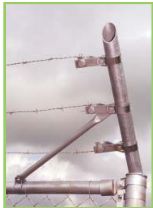
End of run cranked extension detail showing strut
