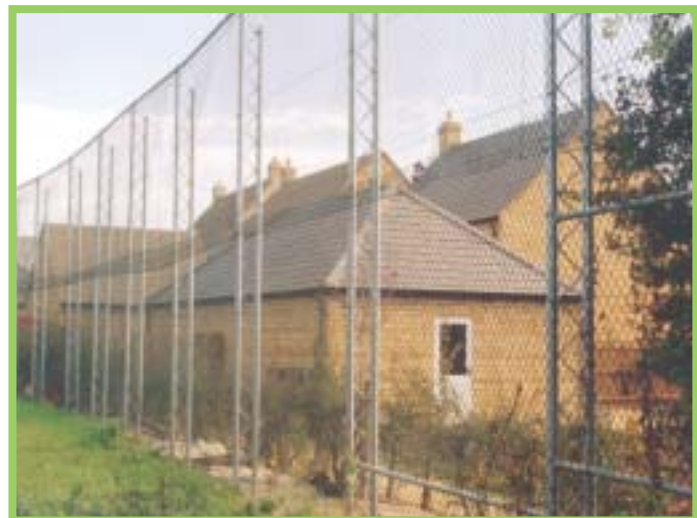
Ball-Stop Sports fencing protecting dwellings at the perimeter of a playing field
