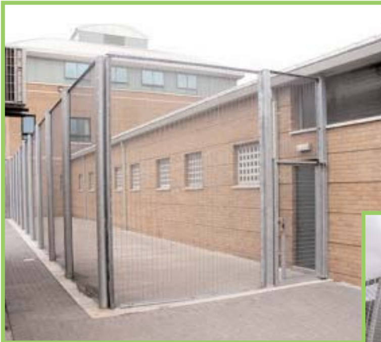
Large single leaf gate with additional Security Comb topping
