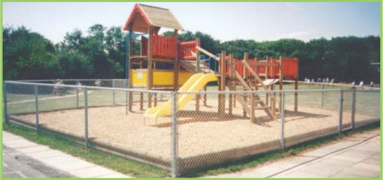
Tubular fencing system of chain link with top rail around playground
