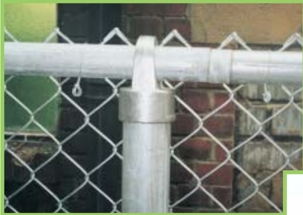
Top rail detail showing connection
