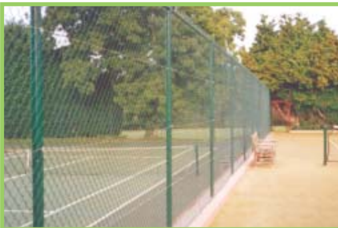
Tennis Court Surround galvanized with polyester powder coated finish clad with PVC coated chain link
