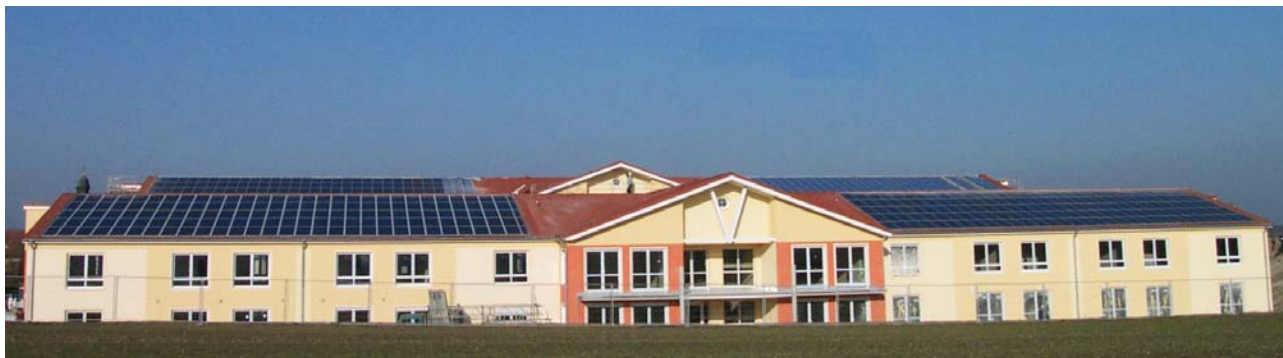
Grid-connected system 130 kW SUNPpower Roof® single crystal modules AS 170
