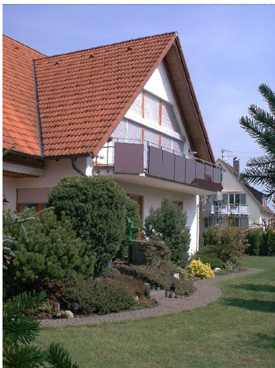
Grid-connected system as a balcony trim amorphous modules KA 60
