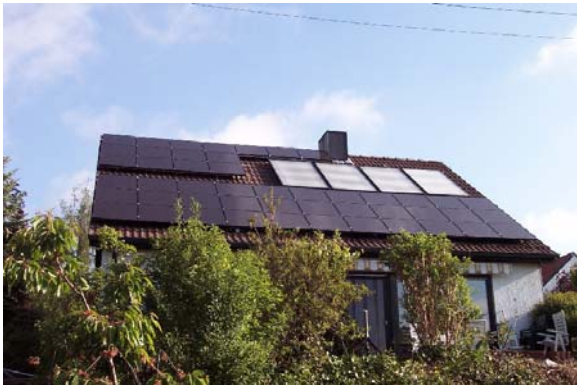
Grid-connected system 5 kW with the module KA 60 and thermal solar system
