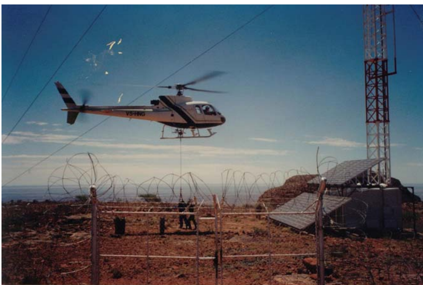
PV-System for a tele- communication system in Southern Afrika
